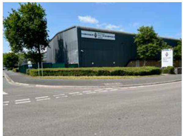
Two storey building with first floor used as open plan offices
