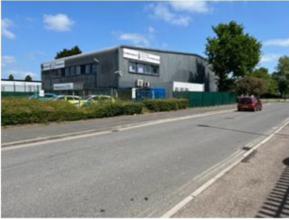
Public Enquiry Office to south west with ancillary buildings housing cycle store & welfare unit
